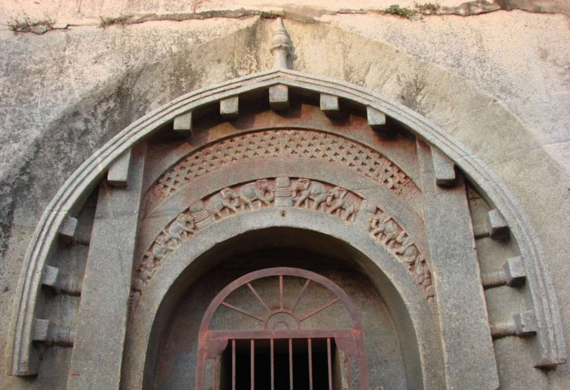
A false arch in the shape of horseshoe, supported by mock corbelling.
