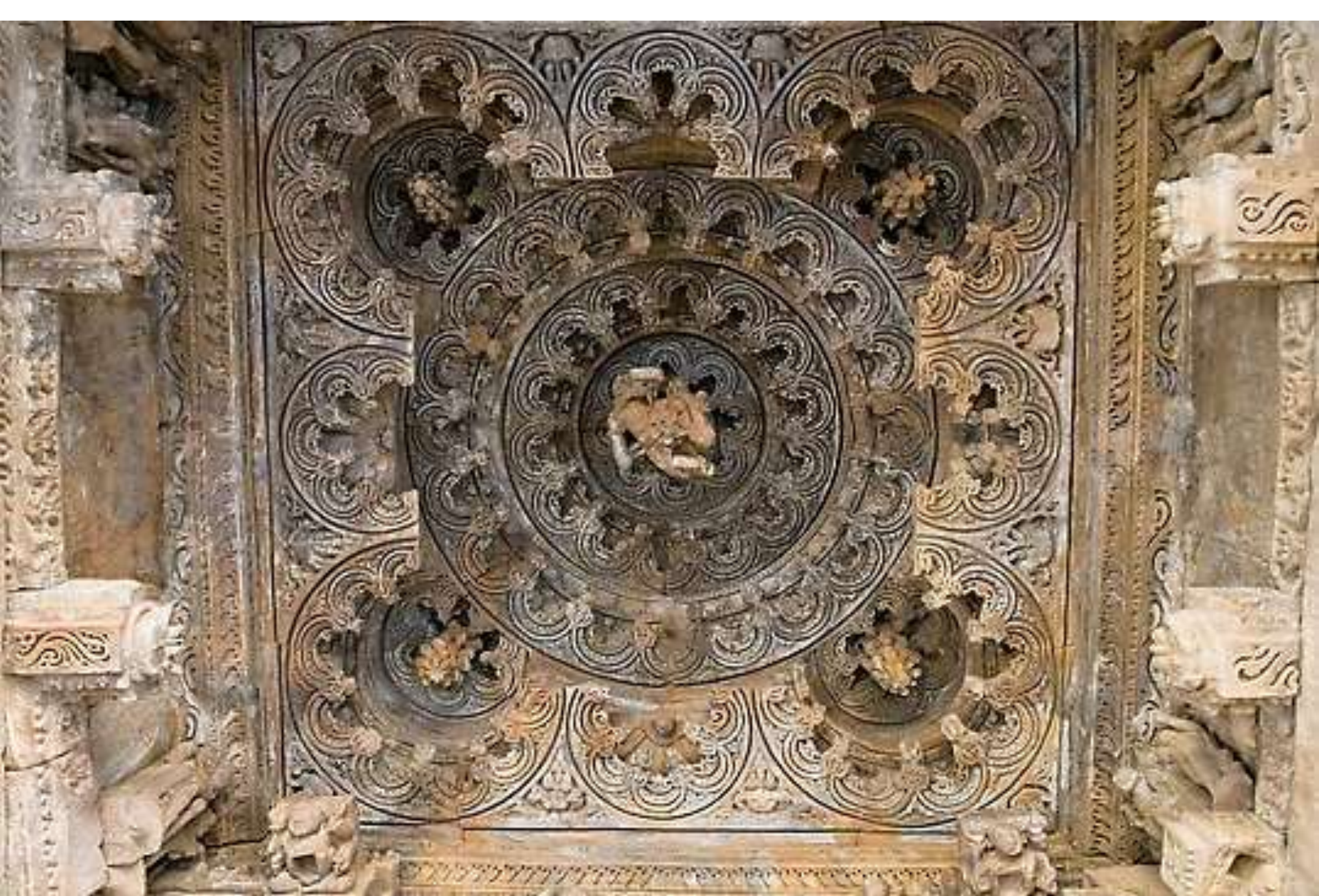
A view of the ceiling
